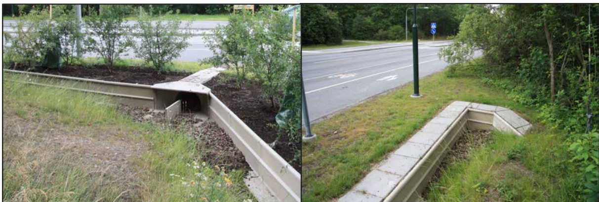
Figure S5. Amphibian tunnel with guiding structure, fence and fence-end at Kyrksjölöten, Sweden. Photo: J.O. Helldin and Erik Jondelius
