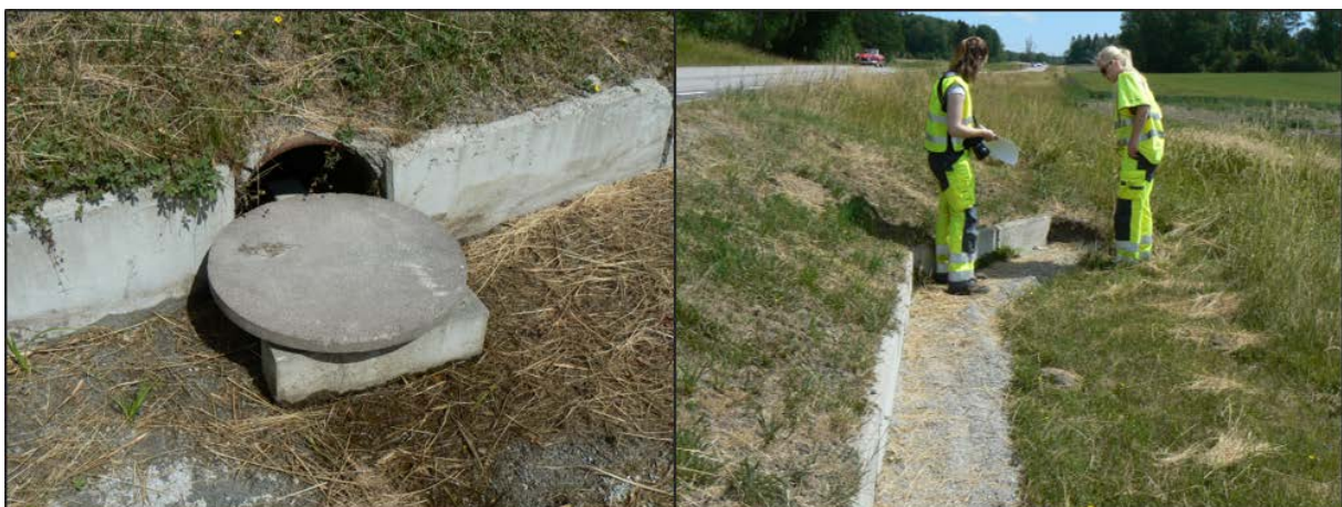
Figure S3. Amphibian tunnel with guiding structure, fence and fence-end at Skårby, Sweden. Photo: J.O. Helldin
